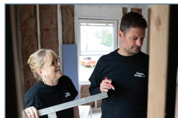
Princeton added interior sheetrock for ceilings and walls for a Habitat for Humanity home in Hightstown.
